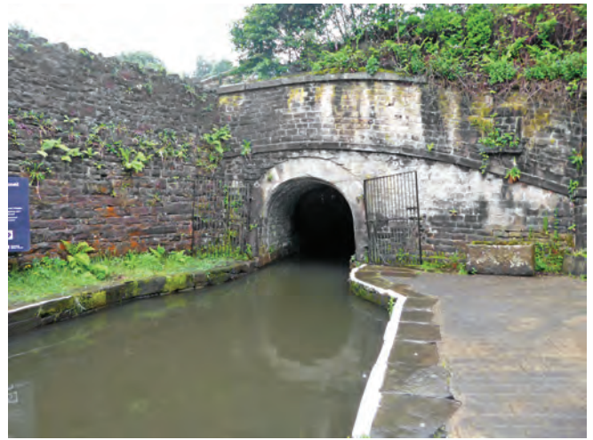
Marsden end portal. Photo Bob Clary
